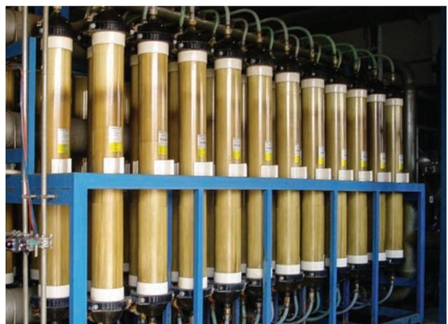
“The most important reason that ultrafiltration was selected for seawater pre-treatment is the high quality of the permeate,” said Mr. Zhang, plant manager. “The high permeate quality results in less frequent RO cleanings and ensures longer RO element life. With the TARGA® II ultrafiltration system, we are able to cost-effectively tap the limitless seawater and avoid draining our scarce surface water resources.”
